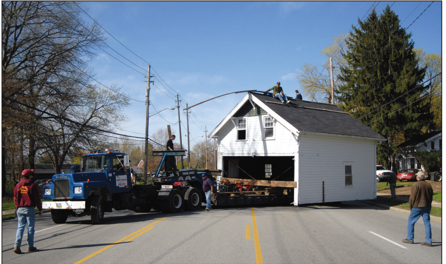
MOVING OUT: Workers guide the old Stearns home on the roadway during its April 19 move to the Olmsted Historical Society's museum campus in the Metroparks. (Photo by Larry Bennet)
