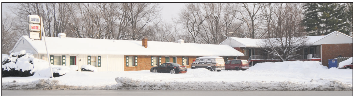
The Cleveland Motel, located at 22735 Lorain Road, will be demolished and the property purchased by the city of Fairview Park. (West Life photo by Larry Bennet)
