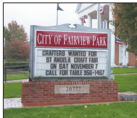
The marquee sign in front of Fairview Park City Hall is broken and needs to be replaced, city officials said. (West Life photo by Kevin Kelley)
